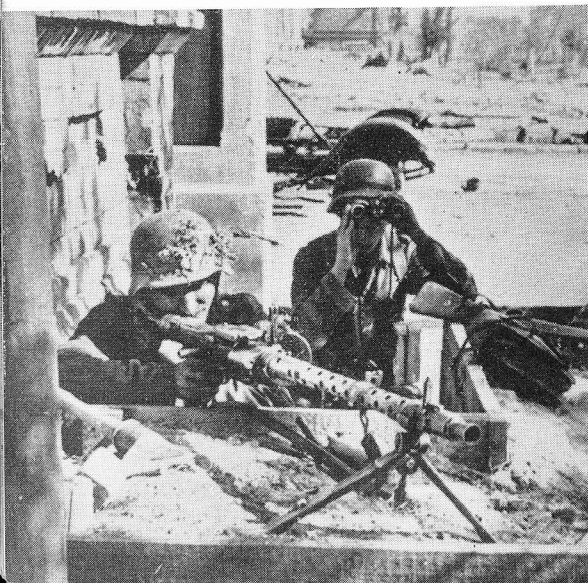
The very efficient MG 34 was the standard machine gun of the Wehrmacht. It had a high cyclic rate of fire and was relatively simple to operate and maintain. It could be used with 50 round belts or 75 round drums in the ground fighting role. In the medium machine gun role (above) it had a crew of five and a tripod mount. There were two of these guns to each of the two medium machine gun sections of the heavy platoon in a rifle company. In the light machine gun role the MG 34 was used on a folding bipod mount in each rifle section (left).
